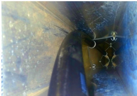
View of vibration dampner inside an aluminum light pole.
