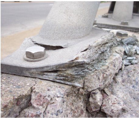
Corrosion at the base of a pole.
