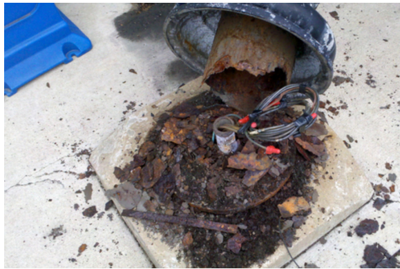
Rust and corrosion inside of a pole.
